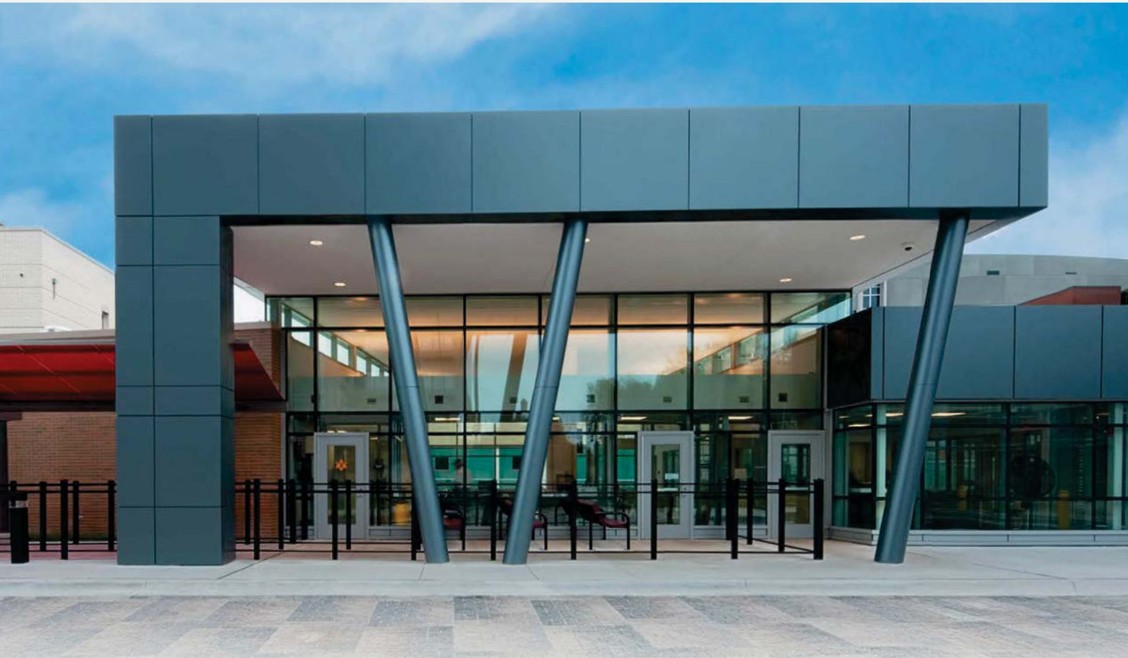
Cook County Jail Complex, Chicago, Illinois (largest jail in country). The buildings screen visitors and employees for contraband materials with metal detectors and drug and x-ray scanners. The main visitor center entrance has exterior canopy for visitors, waiting outside building to be screened; separate fence lines for visitors and employees; inside waiting area for posting bond for detainees; control room for building and parking lots and gun room. On a busy day, over 6,000 visitors are processed at the main building.
