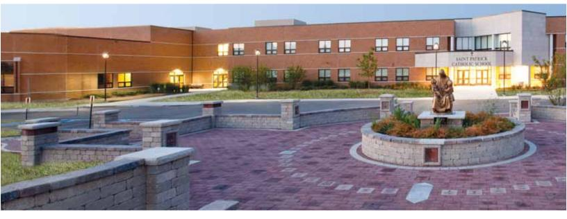
Insulated masonry cavity wall was the system chosen for aesthetics, cost and thermal efficiency. The wall system allowed for a smaller HVAC system to be used, while also providing loadbearing capacity, sound and vibration dampening and increased fire rating.
